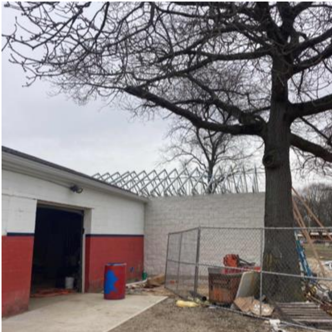
East Field House – Complete masonry, start roof trusses, start and complete concrete walkways around new field house
